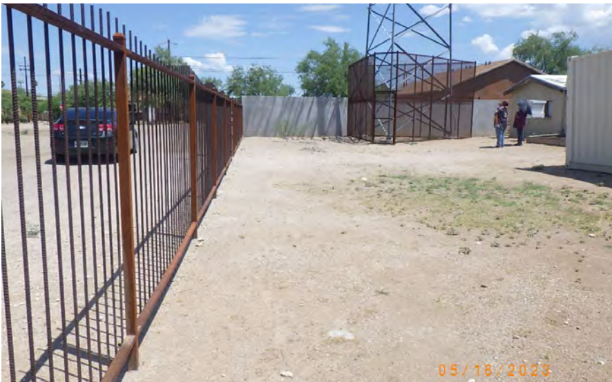
G: Northerly View of the Proposed Fiber Run, Proposed Generator and Propane Pad, Proposed Cabinet, and Proposed Power Route Options
