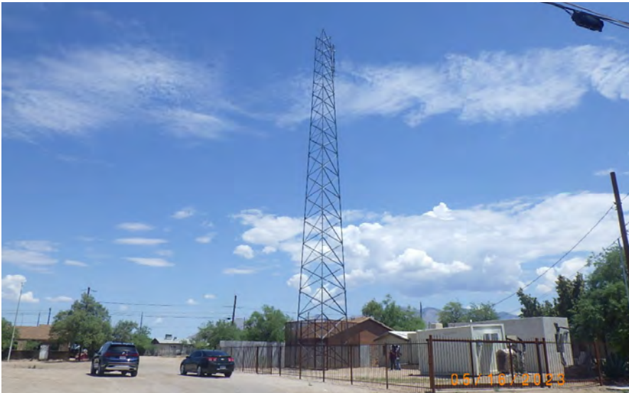
E: Northeasterly Overview of the Existing Tower
