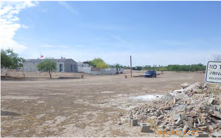
E: Southeasterly Overview of the Proposed Tower Compound
