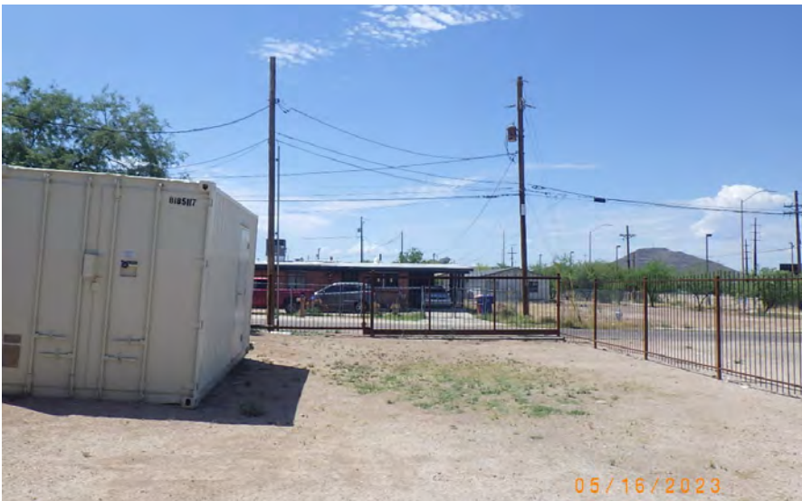
C: Southerly View from the Existing Tower
