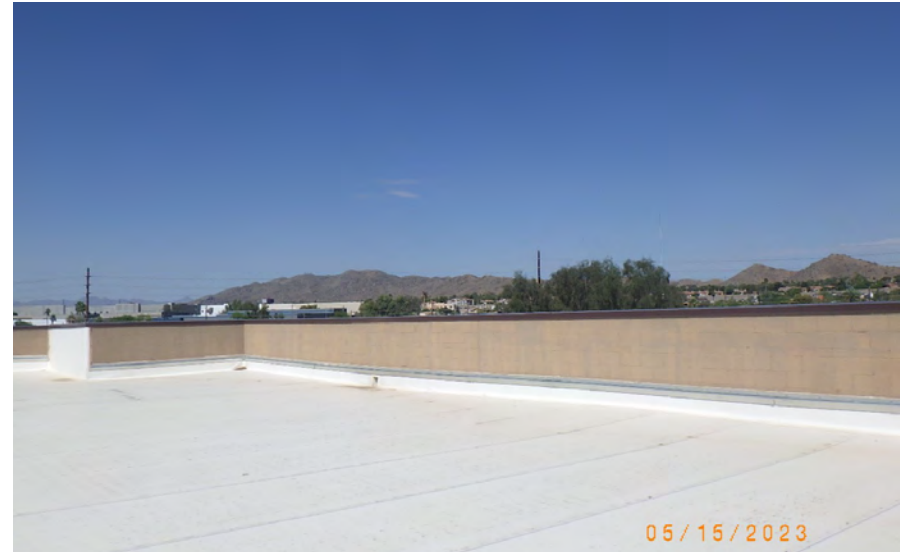
F: Westerly Overview of the Rooftop
