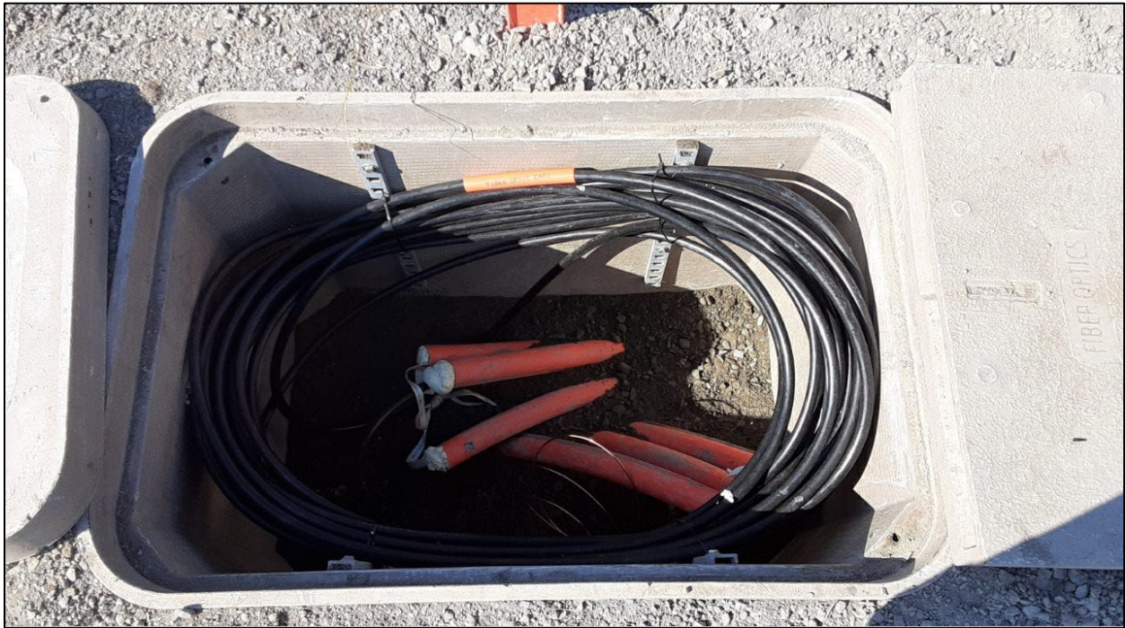
Photograph 4: Typical Vault Buried Flush Following Construction
