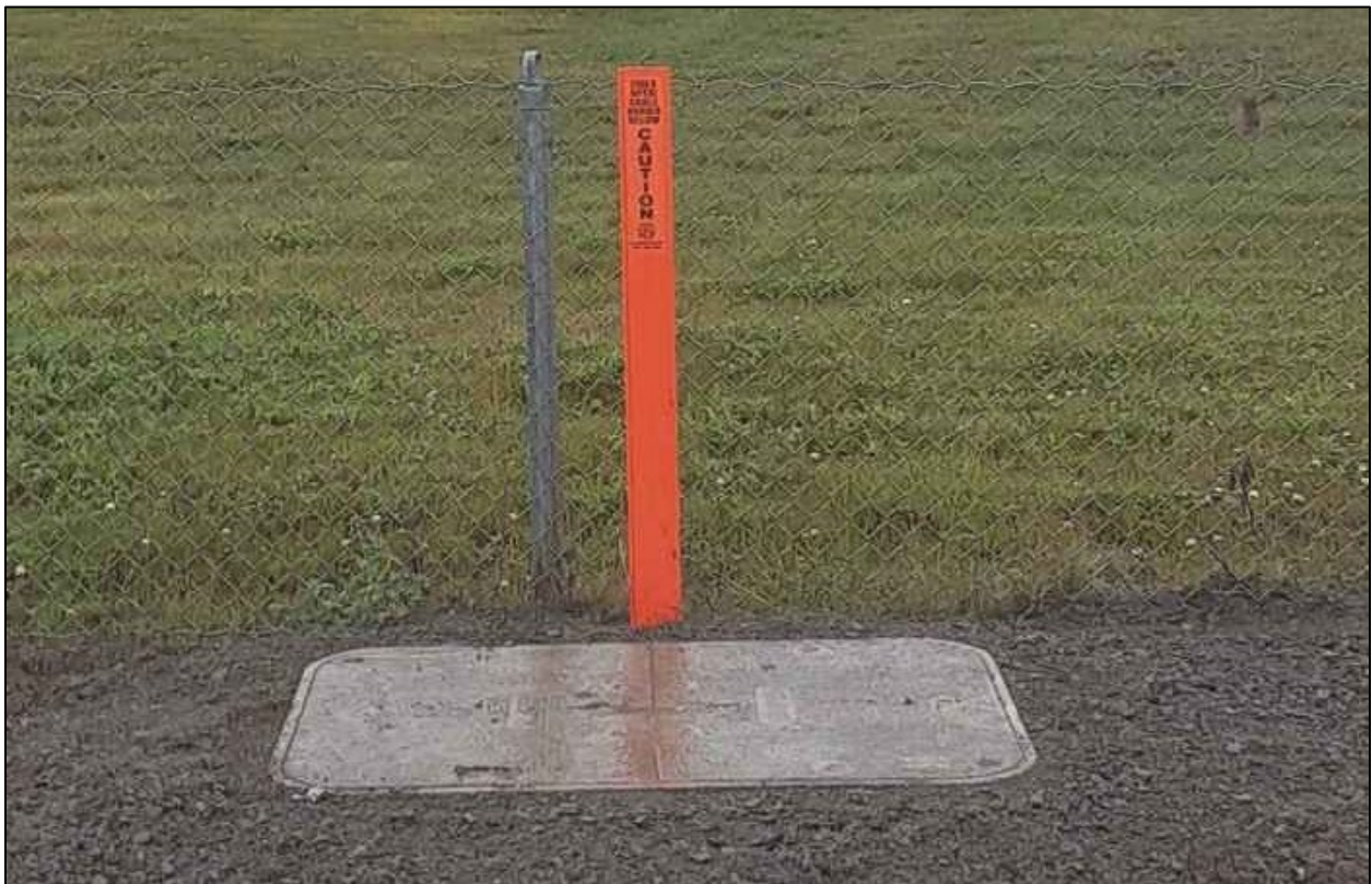
Photograph 4: Typical Vault Buried Flush Following Construction
