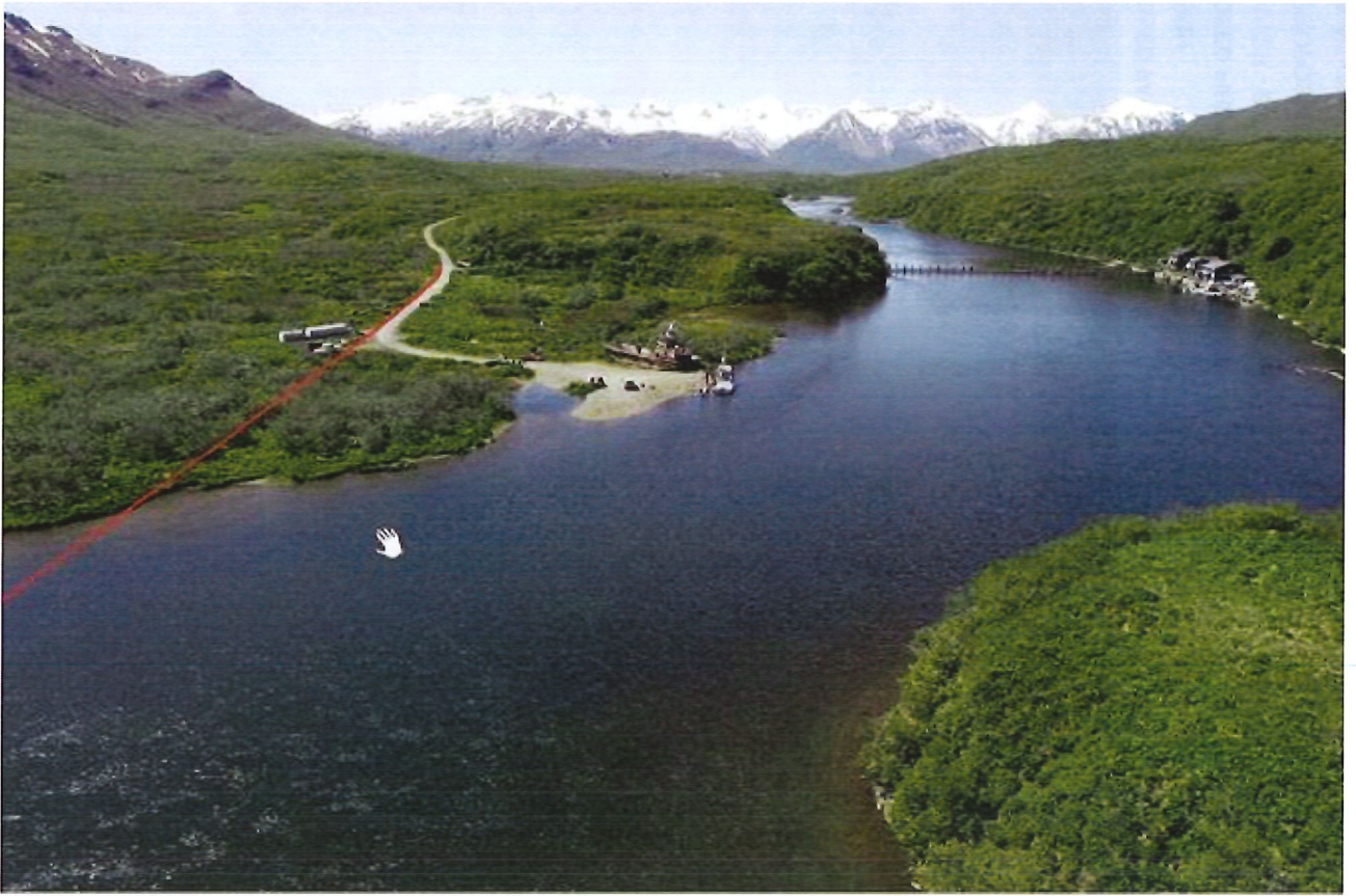
Photo 1. Red line indicates route of the fiber optic cable from the Chignik River to land.
