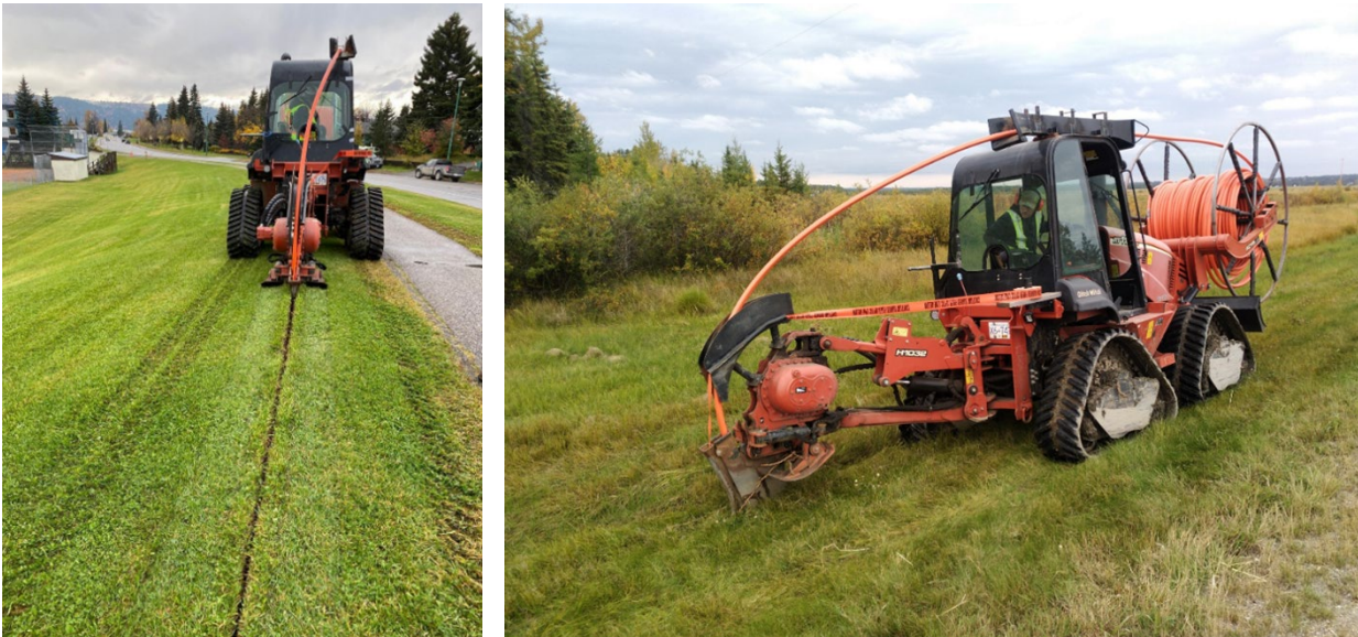
Figure 3. Typical vibratory plow.
