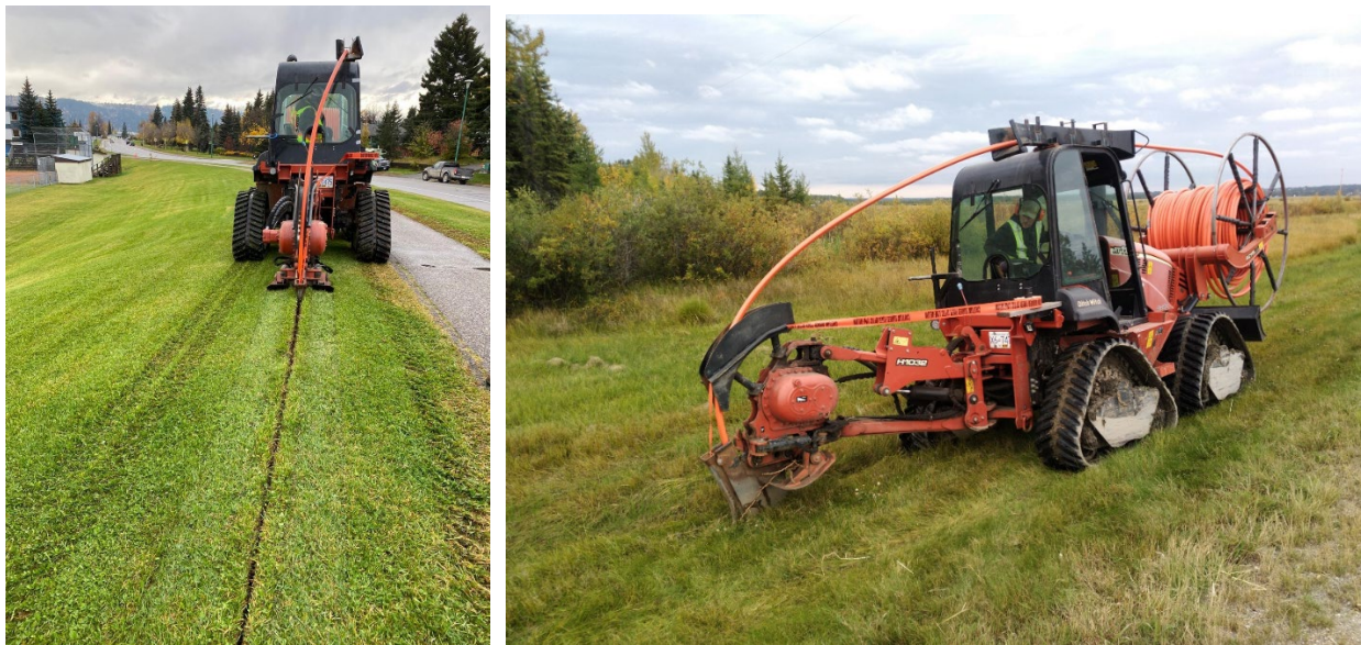
Figure 7. Example of equipment used for FOC installation along the Canyon Bypass.
