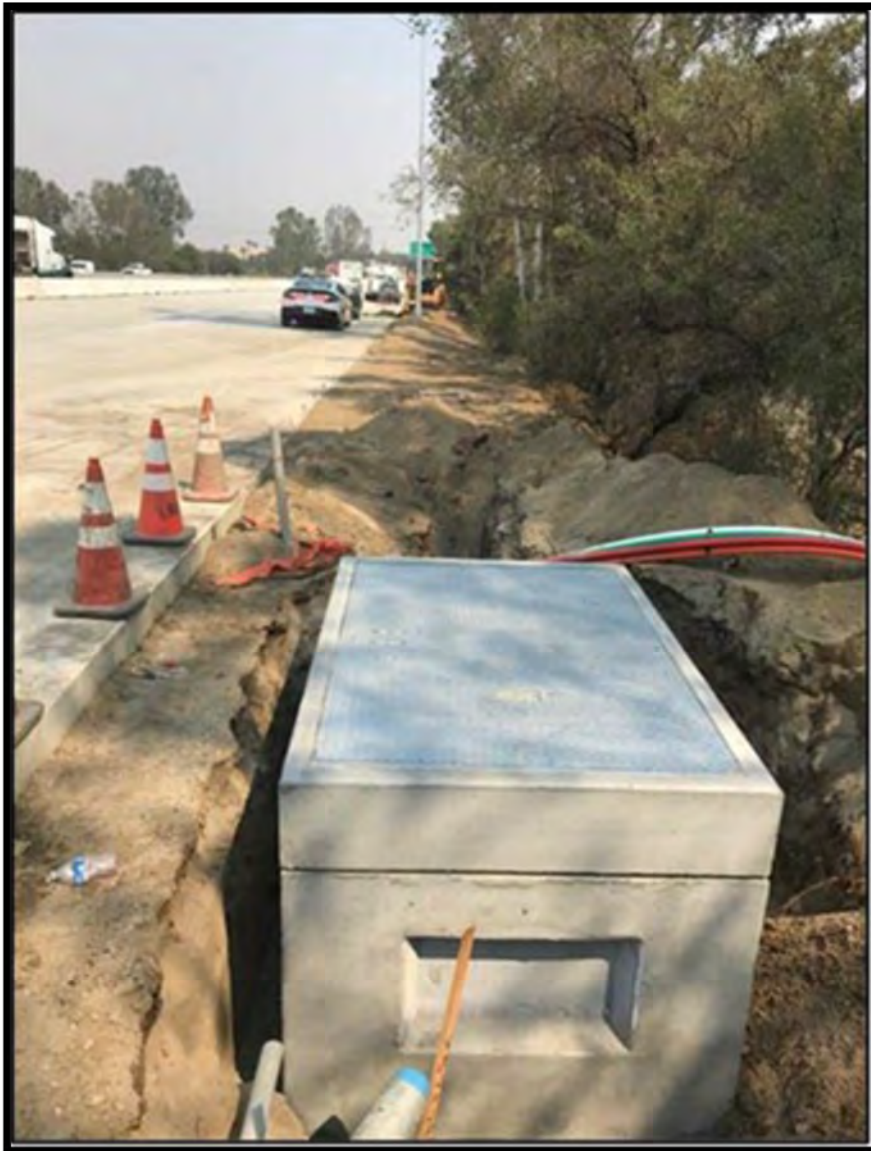
Figure 5. Vault Installation
