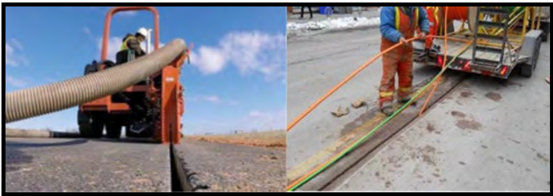
Figure 2. Micro-Trenching
