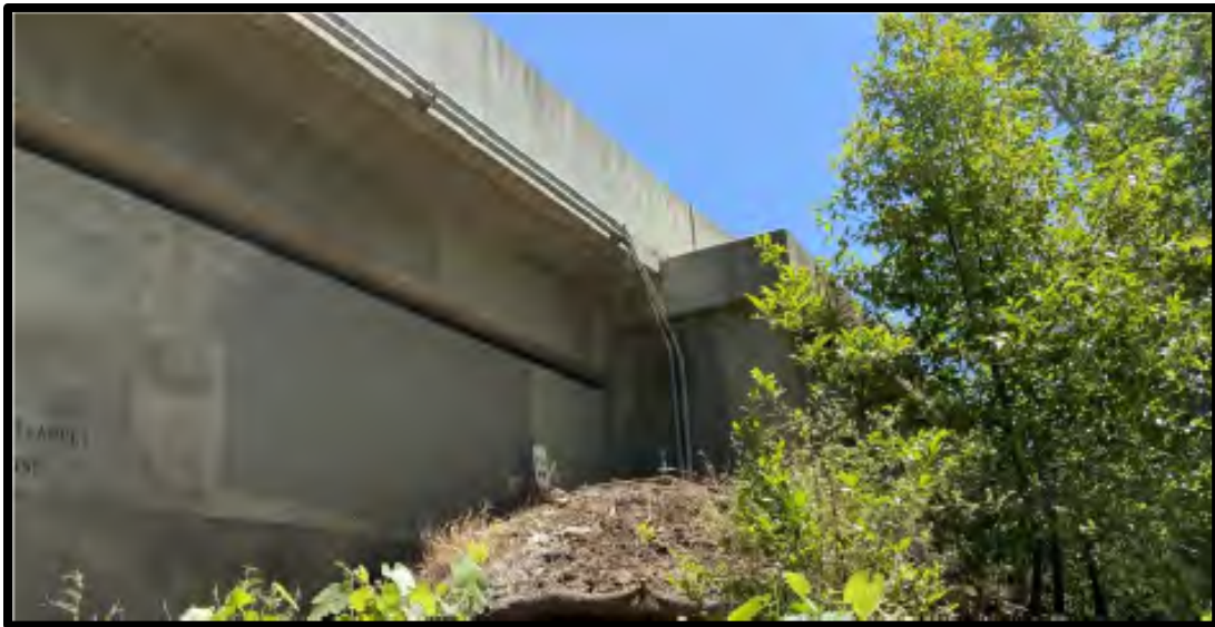
Figure 4. Conduit Attached to Existing Structure
