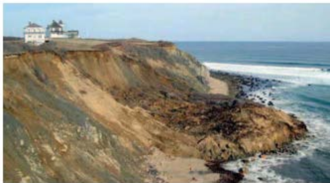
Block Island Bluff Landslide
