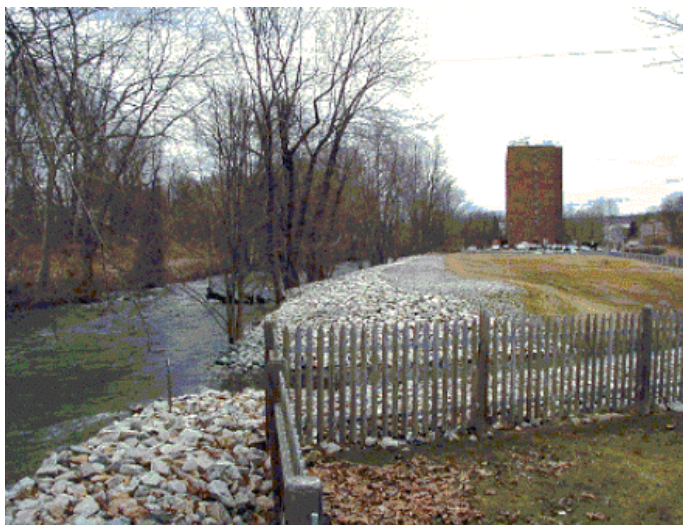
Centredale Manor Restoration Superfund Site
