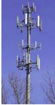
Figure 2.4.3-1: Monopole Cell Tower with Multiple Panel Antennas
