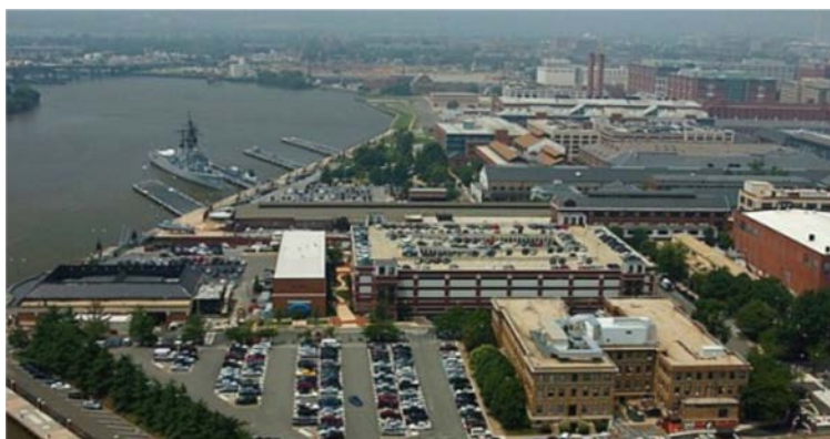
Figure 5.1.15-2: Washington Navy Yard Aerial View, Washington, D.C.
