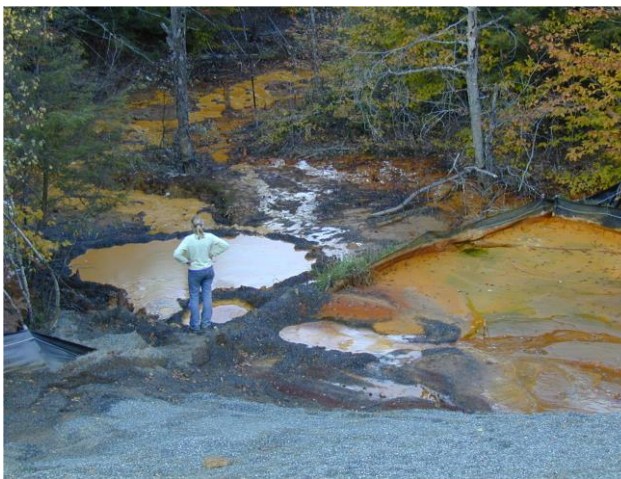
Figure 14.15-3: Iron Seeps Discharging at Base of TP-1, Elizabeth Mine
