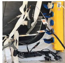
Testing Post Loading
