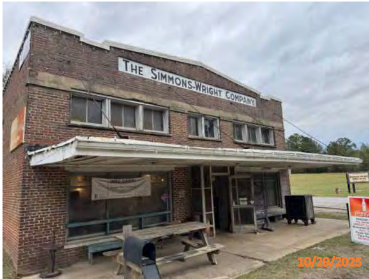
1A: Westerly Overview of Simmons-Wright Company Store (NRHP# 08000198)
