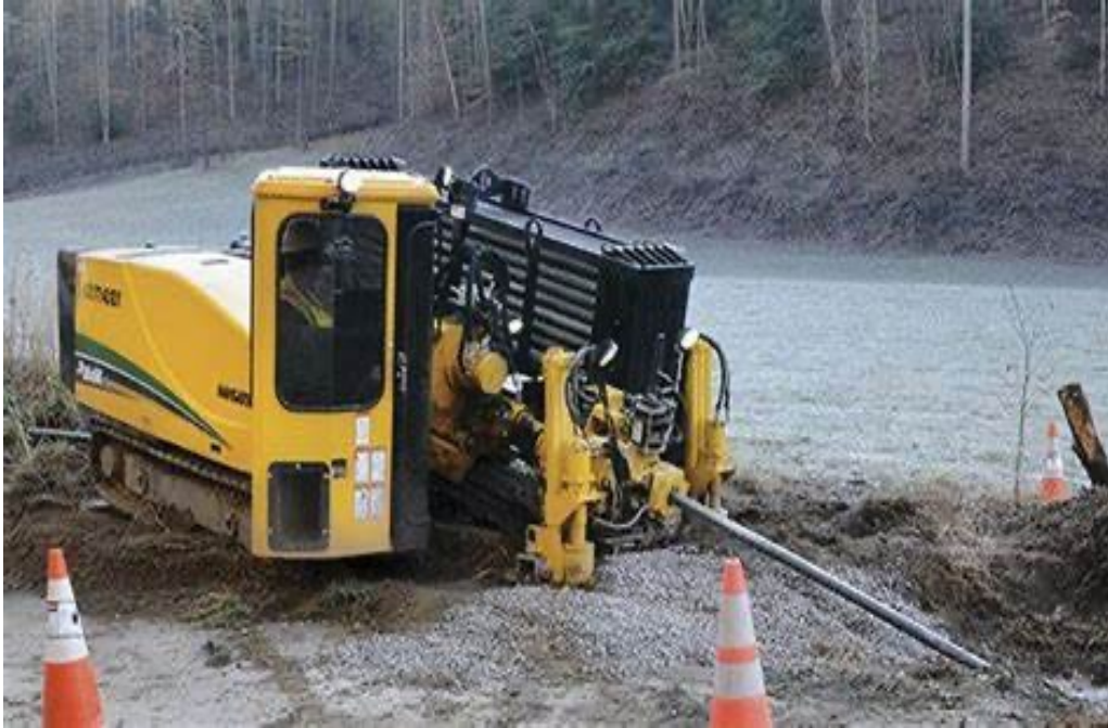
Figure 26: HDD rig utilized in terrestrial boring
