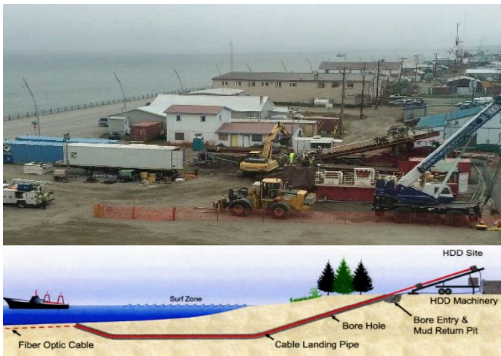
Figure 12: Bore Machine
