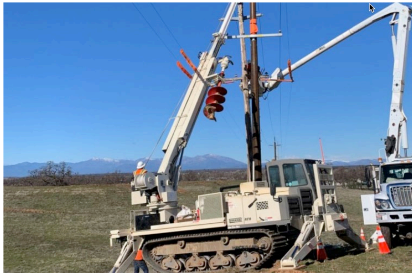
Figure 27: Aerial Pole Construction
