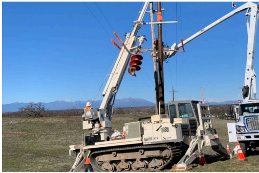
Figure 27: Aerial Pole Construction
